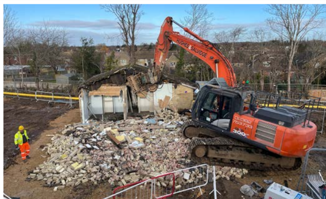
'The Bungalow' under demolition
